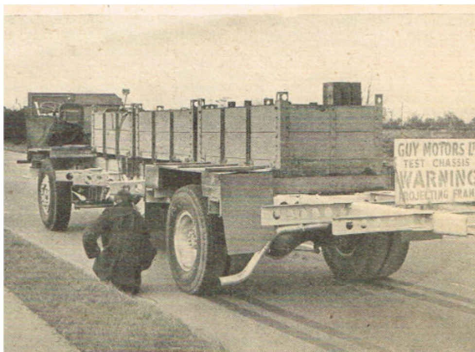
On the 1-8 section of Hermitage Hill, a smooth bottom gear restart was made at about one eighth throttle opening and without clutch slip
