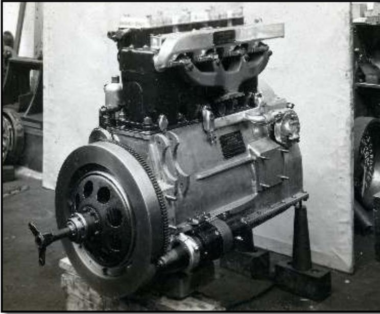
*Given the unusual position of the starter motor, the additional drive from the rear of the camshaft and the drive system from the flywheel it is possible that this is the 4LW that was fitted to the Bentley. The picture's are from an album which is believed to have belonged to Joseph Gardner which also contain's the first 6LW photographs*
