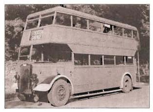
A typical utility double decker. This is 6LW powered Arab Mk.II chasis with a lowbridge body built in Leeds by Charles H Roe
